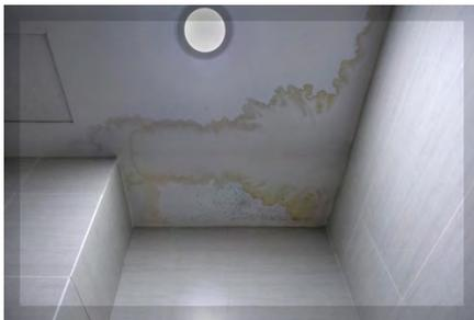
Water intrusion can occur in any type of building - residential or commercial property, hi-rise or a condominium community. It can cause significant damage and lead to a variety of problems, including structural damage, mold growth, and compromised indoor air quality. Understanding the causes of water intrusion and taking preventive measures can help prevent problems from occurring.
